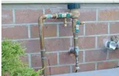
Pressure Vacuum Breaker Assembly Principle Preventer
